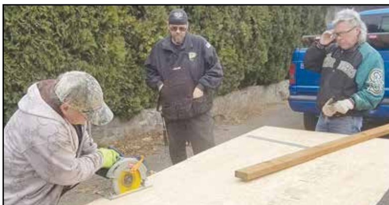
In Spokane, Denny Empson, Jerry Purser and Tony Wade cut wood for the ramp.
