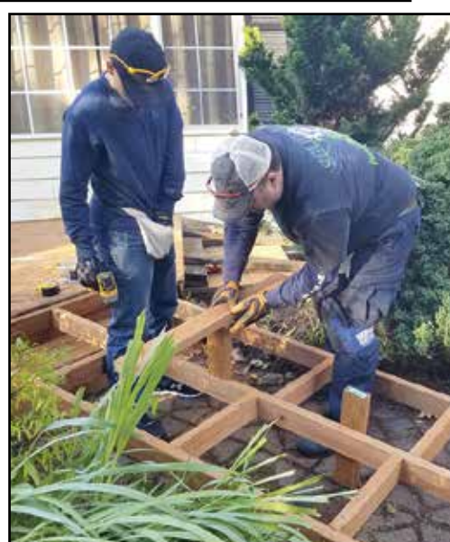
Above: Framing the Tacoma ramp to ensure a gradual decline.
