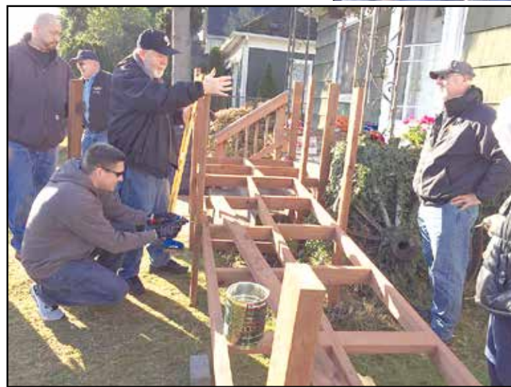
Above: Framing the Tacoma ramp to ensure a gradual decline.
